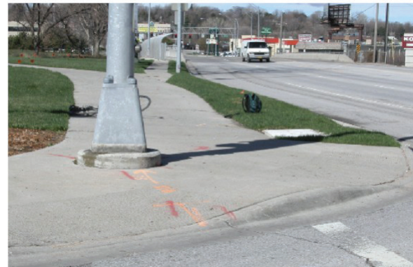
Poor Sidepath Intersection Design. Top: Ramps are narrow and located off line from a bicyclist's normal path, creating a potential hazard. Above: The base of a signal mast arm obstructs the logical path through the ramp.
