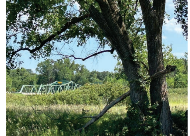
View of the Highway 281 Bridge from pond area
