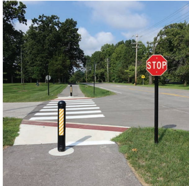
Sidepath with well-marked crossing, Clayton Road in Saint Louis County, MO
