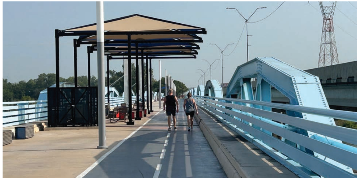
Harmony Bridge, Bixby, OK. This historic bridge with a parallel new highway bridge has been converted into a community park with a shared use path and themes around music and art.
