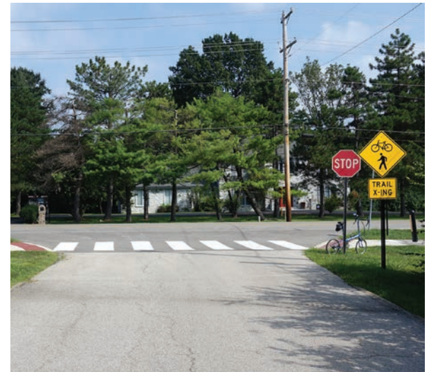
Sidepath Advisory Signs. Top: Variation of the MUTCD's Railroad Advance Warning Sign, modified as a sidepath advisory. This sign should be used on both sides of a road with sidepaths. This installation is on Speer Boulevard in Denver, advising of the parallel Cherry Creek Trail. Florida DOT advises a similar sign. Below: Trail crossing advisory sign on an intersecting side street, installed on Clayton Road in suburban Saint Louis.
