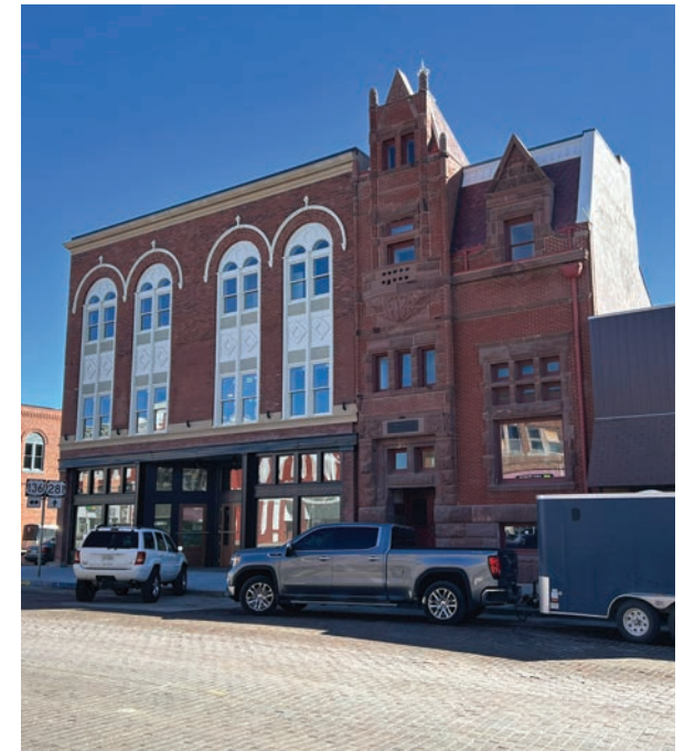
Hotel Garber. This superb boutique hotel was developed largely with private philanthropic funds for the purpose of increasing tourism in Red Cloud. It demonstrates the commitment of Nebraskans to Red Cloud and the national interest in pioneer history.
