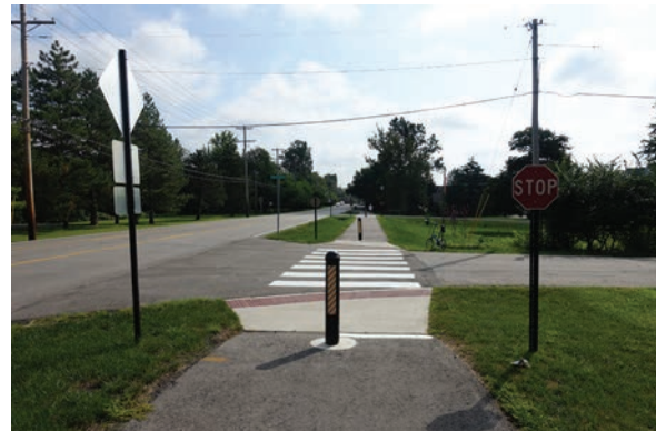
Good sidepath intersection design: Ramp is directly in line with travel path, crosswalk is unobstructed and clearly marked.
